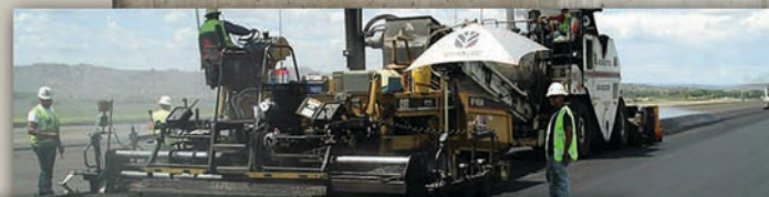
Asphalt and Paving
