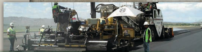
Asphalt and Paving
